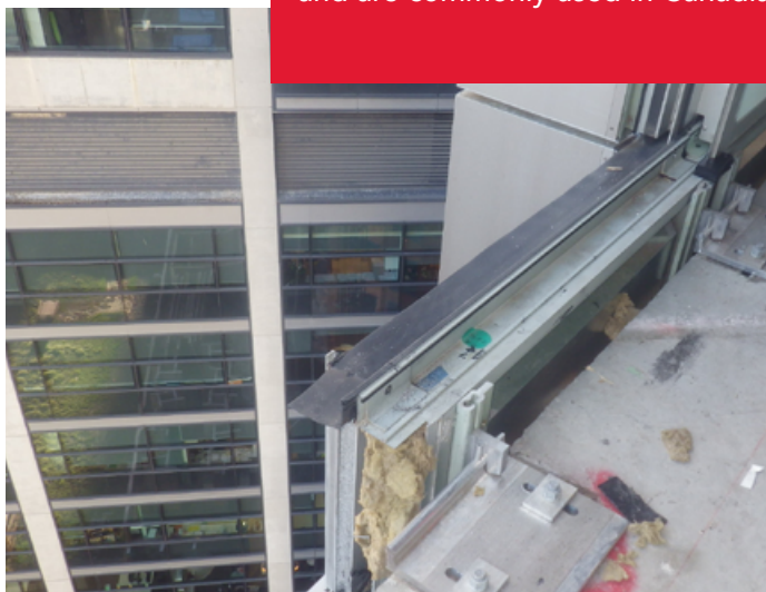
Stone wool insulation being installed as part of a curtain wall firestopping system
